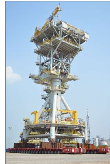
Mooring Tower – fabricated by BMI for Mobil CEPU, installed at Java Sea (36km North of Tuban).
